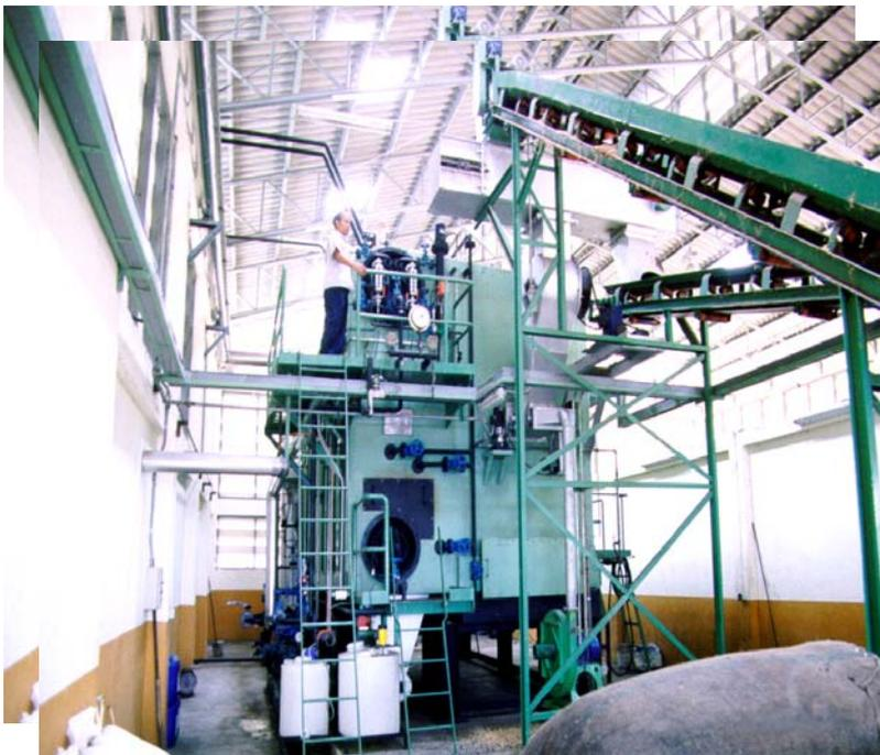
Fluidized bed Boiler for Superheated Steam Production
